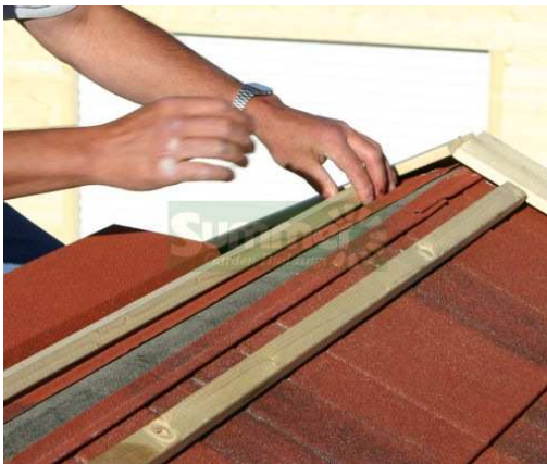
Close up view of the ridge tiles and battens
