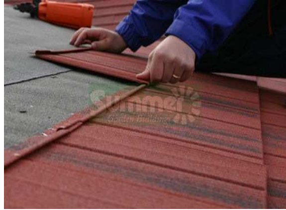
Fitting the granular steel tiles
