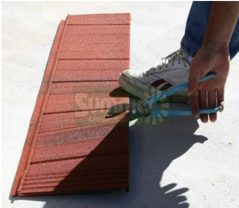
The tiles can be cut with snips or a hacksaw
