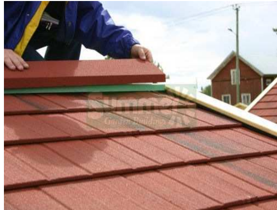
The final ridge cover being fitted
