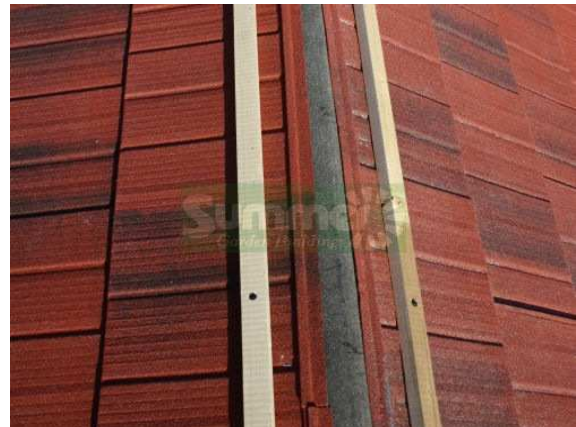
The ridge tiles and battens viewed from above
